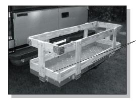
4. Attach the "bottom layer" 1x4's to the upright 24" posts previously installed. Boards should be centered so that there is equal spacing on each end. Use two #8 1-1/4" wood screws at each post.
